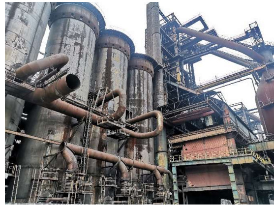
Figure 2: Dolní Vítkovice - historical industry park in Ostrava
