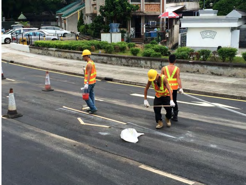
Figure 13: Workers are pasting adhesive tape for road markings
