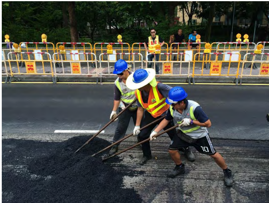
Figure 12: New asphalt is being poured and distributed by workers
