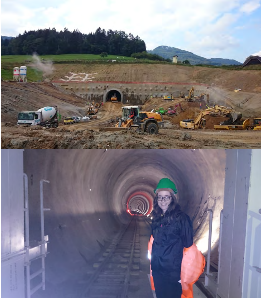
Figure 1: Tunnel construction site visit
