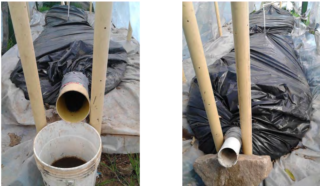
Figure 23: Inlet (left) and outlet (right) of the bioreactor
