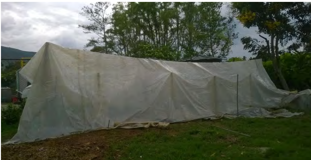
Figure 20: Improvised roof construction.
